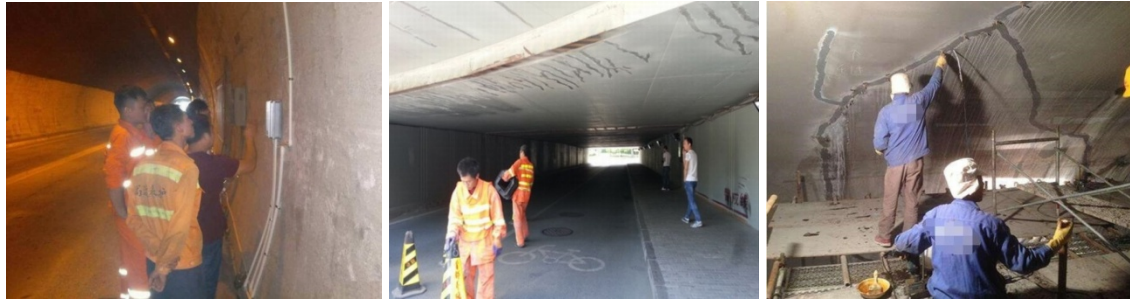
Figure 2. Traditional testing and repairing method
