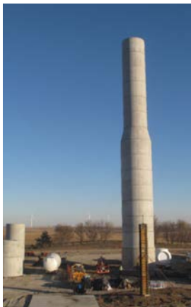
Iowa has the tallest land-based (US) wind turbine (115 meter hub height) Donnelle Eller
