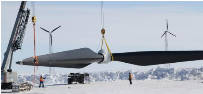
Blade installation in Kotezebue Alaska, used with permission KEA
