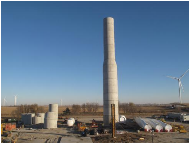
MidAmerican building tallest land-based (US) wind turbine (115 meter hub height) Donnelle Eller
