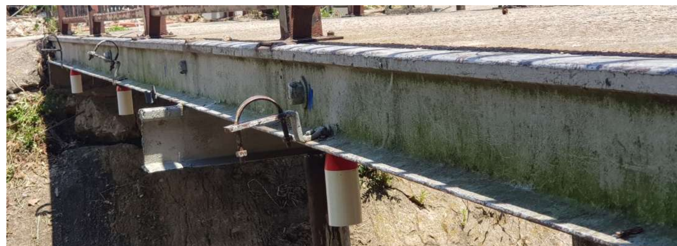
EMP engaged and attached to underside of pedestrian bridge.
