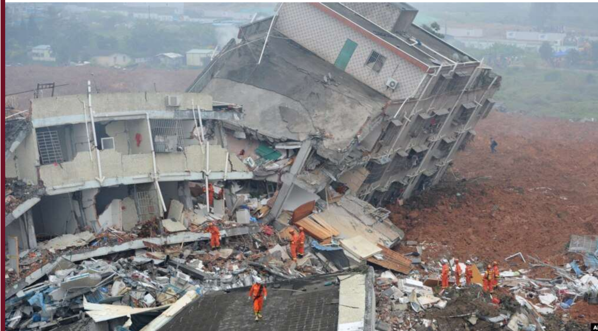
Figure shows unstable building after a landslide compromises its structural integrity.
