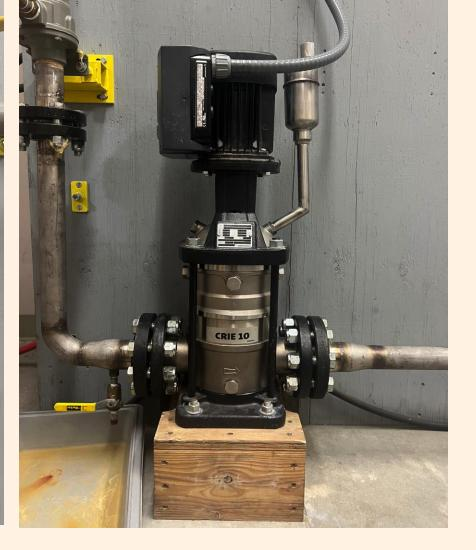
Our system is first filled up with water then the pump Fig. 3) rotates the water through the pipes to get rid of as much air as possible. Then the valves (Fig. 2) direct where the water fill, we leave these open as the SMR is turned on. In Fig. 2, we have the heat pipe generates heat as water circulates through the system. This water increases from 25 C° to around 40 C° while the SMR runs for about three hours.
