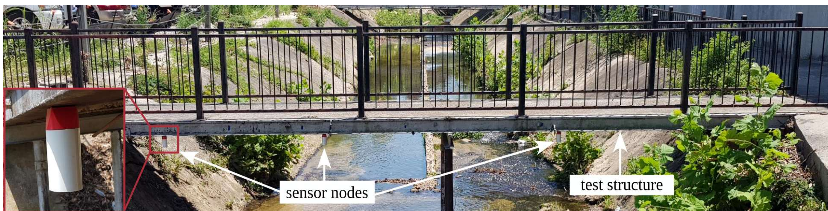
SHM sensing node deployment
