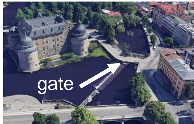
Photos of the flood gate by Austin Downey in Örebro Sweden, Creative Commons BY-SA 4.0. 3D view taken from Google Maps in October 2024; copyright held by Google.
