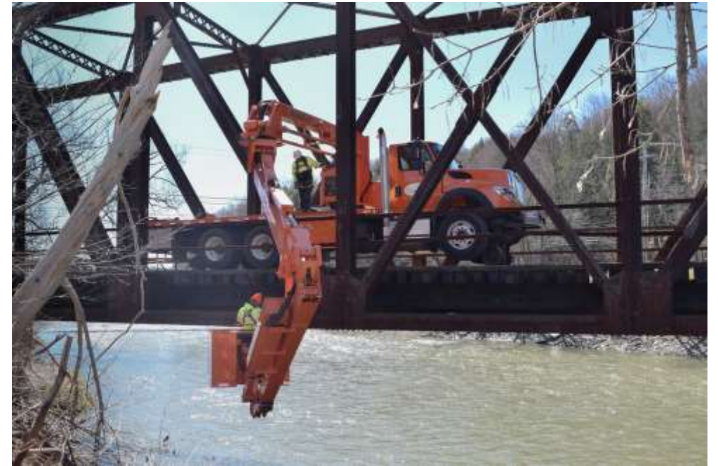
VTrans Rail Bridge Inspection Public Domain
