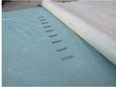
Figure 2 Attaching solar cells and laying down the glass fiber CSM
